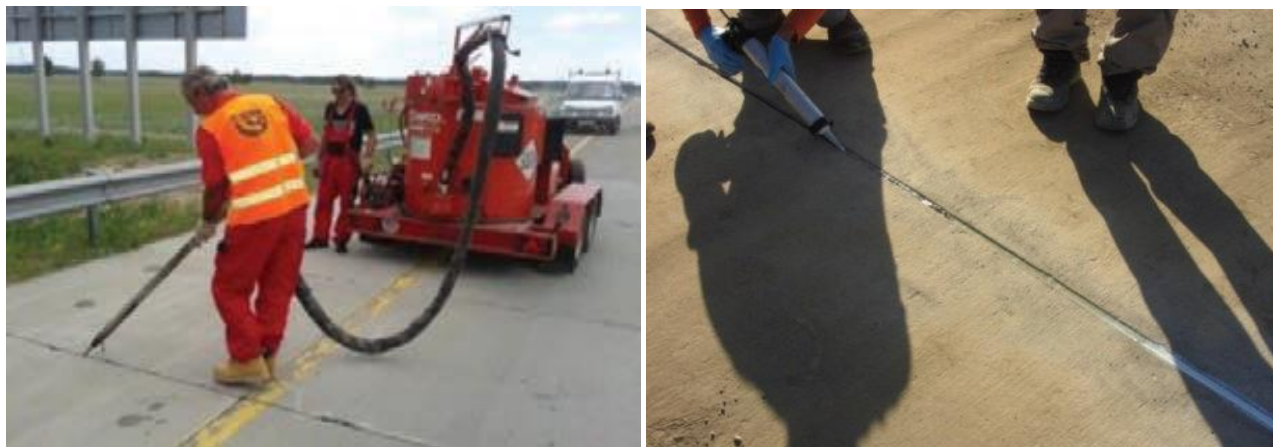
5-rasm: “BIGUMA” mastikasi va “Masterflex-472” germetigini o‘rnatish texnologiyasi
