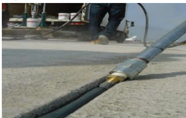
6-rasm: "Crafcro Road Saver" silikonli germetigi va "CRAFCO" polimer bitumli mastikasi
